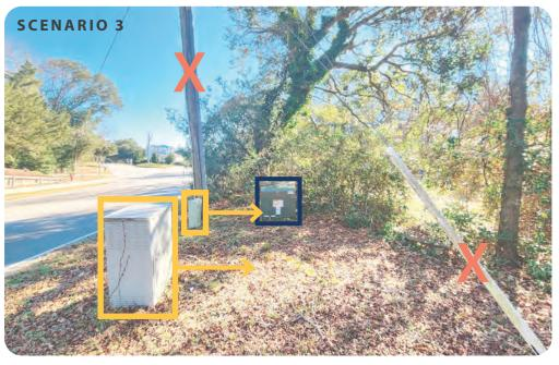
Utility relocation where both pedestals shift westward, indicated in yellow. The transformer, indicated in navy, is not expected to be a conflict for the trail and will remain in place. The utility pole and guide wire are removed. The trail alignment stays close to the road. One of the two preferred scenarios for adjacent property owners.
