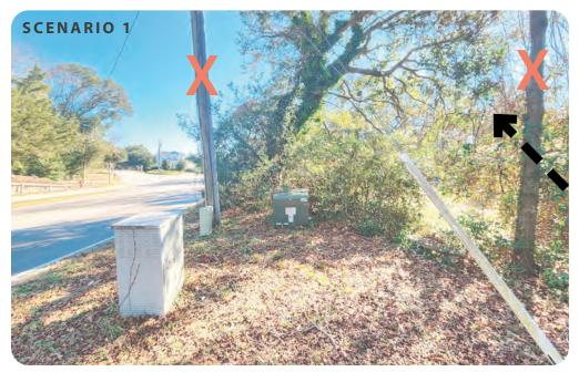
Utilities remain in place, avoiding the right-of-way conflicts by using an easement for the trail alignment, indicated in black. In this scenario several trees and shrubs are removed.
