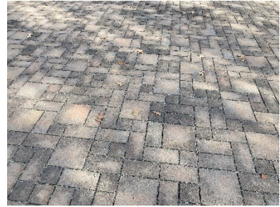
Example of Permeable Concrete Pavers used for a Parking Lot
