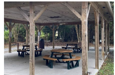
Example of Existing Composite Tables over Concrete Surface at Duck Town Park
